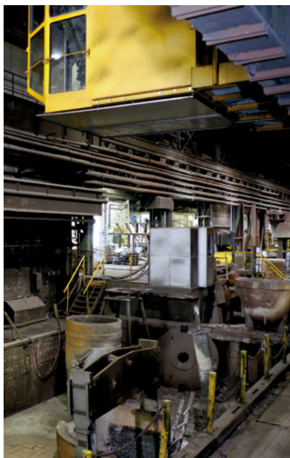
The crane driver in the control cabin (top right) sees all the temperatures of the relevant ladles
