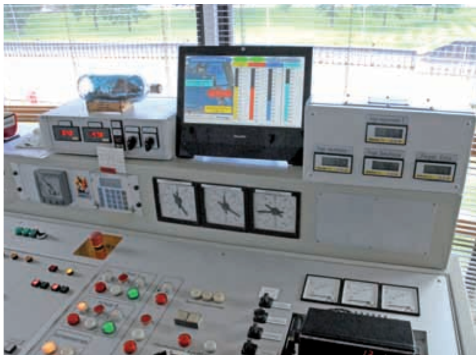
At a glance: The display at the central station always shows the water level of the Ems, the lock and both inner harbors
