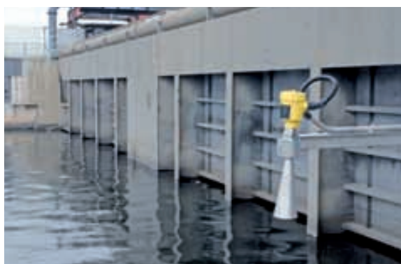
The waves of the radar sensors are reflected by the water surface, the elapsed time defines the level
