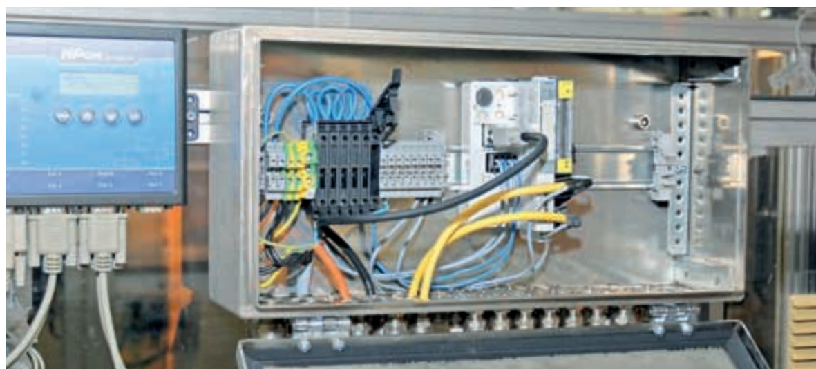
The BL20 gateway is programmable with CoDeSys and carries out the RFID communication
