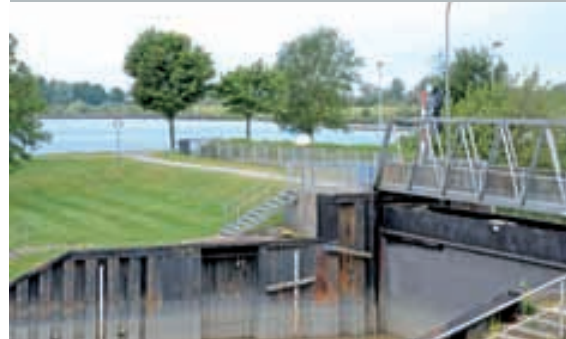
Turck's DX70 guarantees an efficient, wireless data-transfer of the water level measurement at the sea and domestic port in Papenburg. Page 28
