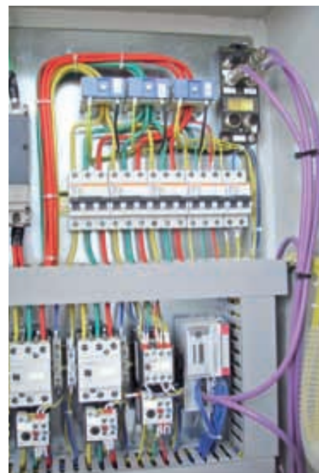
BL20 station and Profibus repeater
